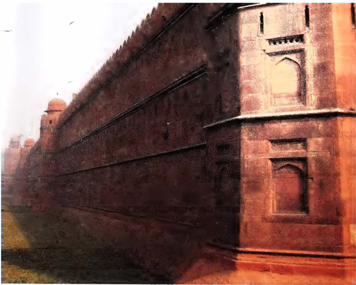
FIGURE 1 Part of the walls of the Mughal Empire's massive Red Fort in Delhi (2012).
